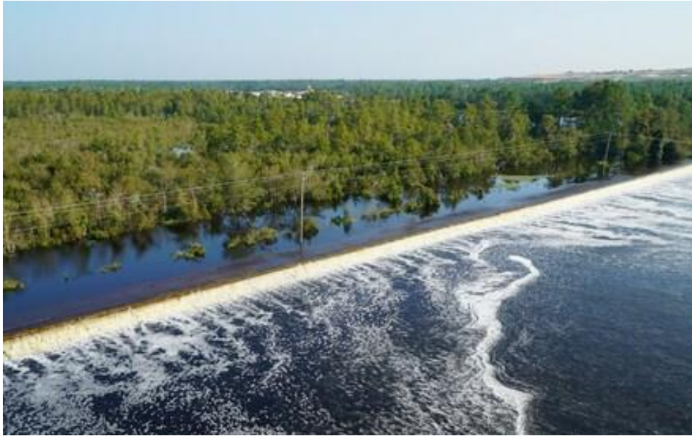
Photograph released by Duke Energy shows flooding from the swollen Cape Fear River overtopping an earthen dike at the L.V. Sutton Power Station near Wilmington, NC. (Washington Post, September 22, 2018)
